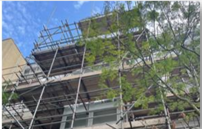
Photo showing Phase 2 North Elevation scaffolding installation works progressing
