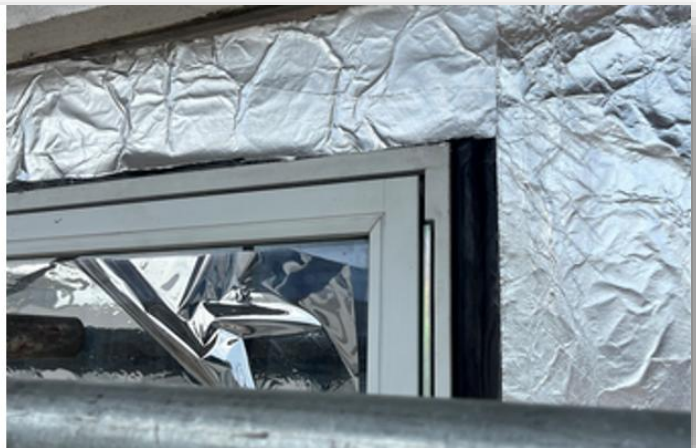
A photo showing Phase 1 South Elevation – New Obex Breather membrane installation works Progressing
