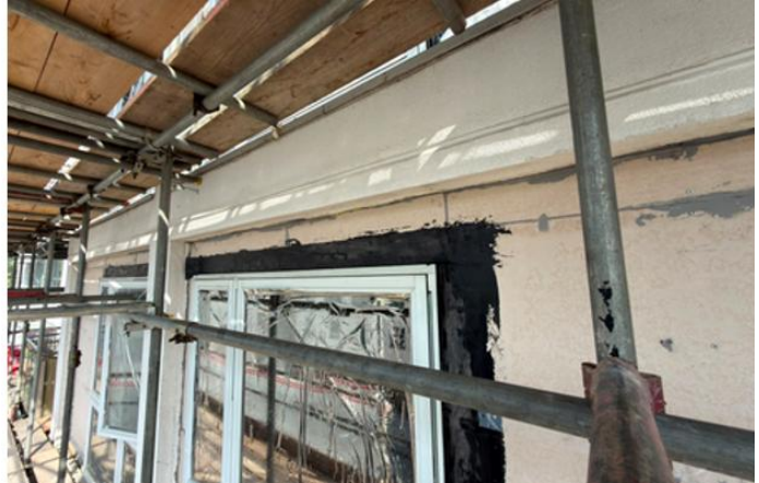
A photo showing Phase 1 South Elevation – New Obex sealing membrane installation works progressing
