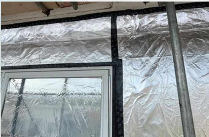
A photo showing Phase 1 South Elevation – New Obex Breather membrane installation works progressing
